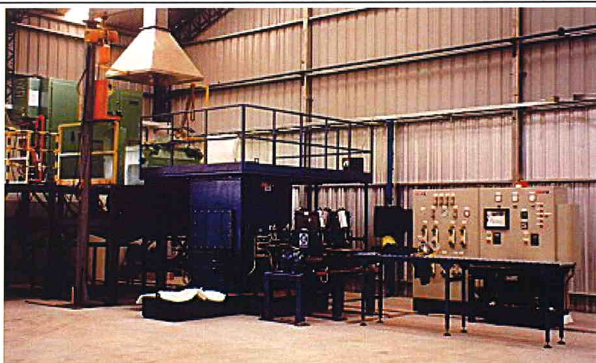
Fig 7 Induction Premelting and RT850 Installation
